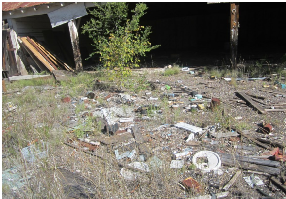
PHOTOGRAPH No. 24 Debris in unpaved area between main maintenance and garage buildings.
