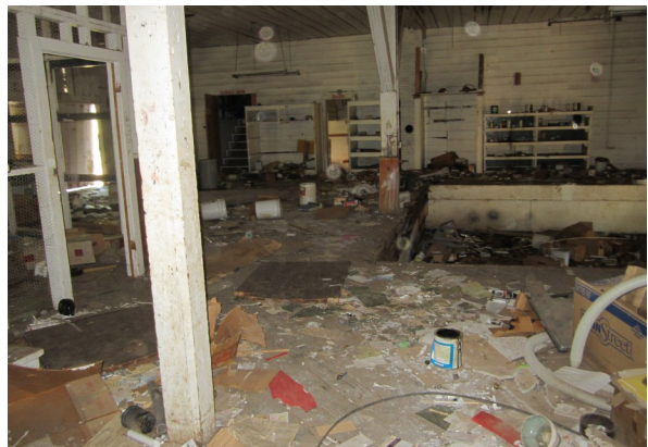
PHOTOGRAPH No. 25 View of paint shop in main maintenance building.
